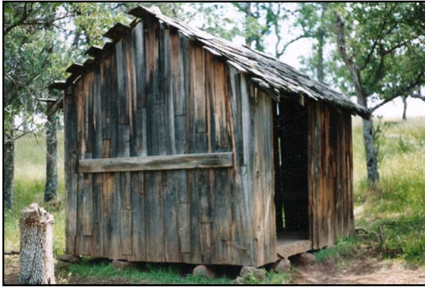
Figure 360. The Robert E. Ward "Line Cabin" on the old Lassen Emigrants' Trail, built in about 1955 by Robert E. Ward, now deceased. This structure has the attributes of line cabins of yesterday, namely, its wooden floor, the foot stones, its board and batten wall construction, and its roof covering of sugar pine shake shingles. Photograph by author, 5/07/2005.
