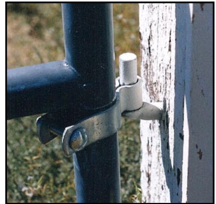
Figure 421. This is a typical lower gate hinge that hangs by gravity. It is on a ranch today in Lassen County. The male bolt part through the "eye" on which the other part turns, is called the pintle. Photo by author, 2007.
