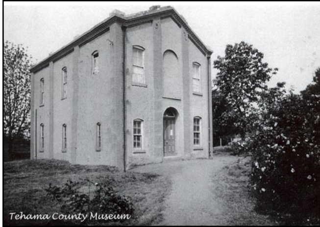
Figure 342. Masonic Molino Lodge #150 of Free and Accepted Masons (upstairs) and Tehama School (downstairs in 1859. The original construction involved 136,508 bricks! (See same structure about one year later, Fig. 90 in Ch. 2, page 137). This building is still extant and serves today as the Tehama County Museum, City of Tehama.
