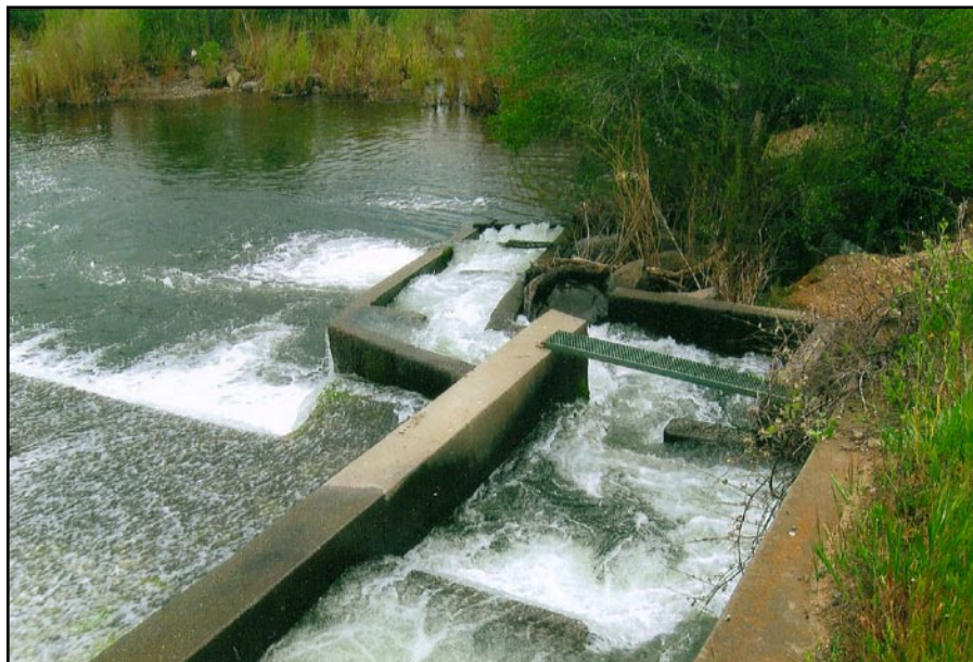
Figure 131. Fish Ladder at lower Deer Creek Dam, Vina, California, part of the Stanford- Vina Irrigation District, Tehama County, to accommodate the anadromous Fall-run of Chinook Salmon and Spring-run Chinook Salmon and Steelhead Trout. Photo taken by author on April 5, 2008.
