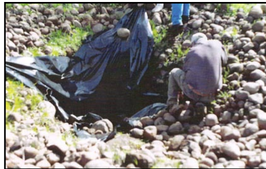
#12 Figure 335. Black plastic tarp cover being placed at bottom of excavating efforts. Photo taken by author on February 28, 2004.
